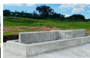
Cattle Trough construction – Tiring’ati Bunda
