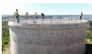
500m3 Kong Hill Tank – Installation of Guard Rails
