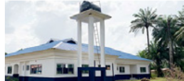
The completed site in Lokomasama.
