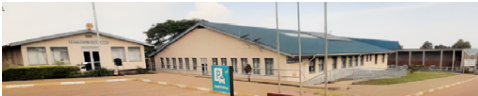
The completed site of the Hospital
