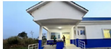
The completed site in PortLoko.
