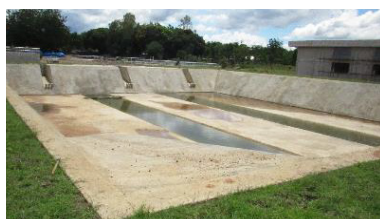
Low Lift Pump station and Sludge Drying Beds
