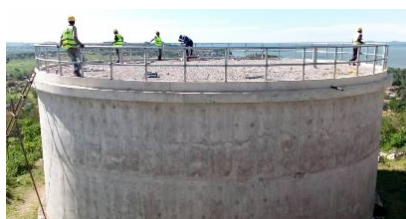
500m 3 Kong Hill Tank – Installation of Guard Rails
