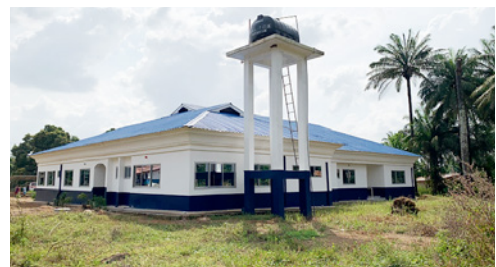
The completed site in PortLoko.
