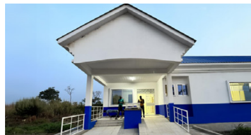
The completed site in Lokomasama.
