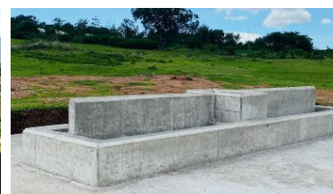
Cattle Trough construction – Tiring'ati Bunda
