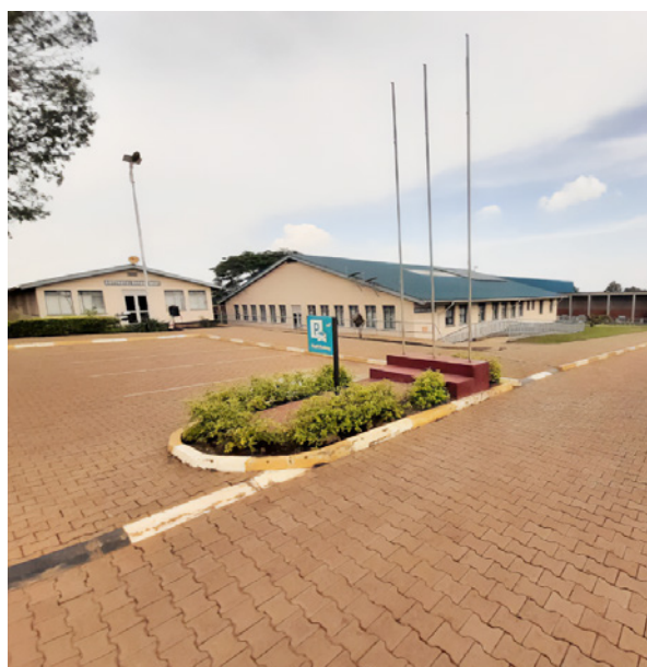
The completed site of the Hospital
